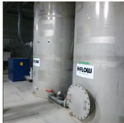
BIOWATER CMFF Bioreactor Units and Blowers
